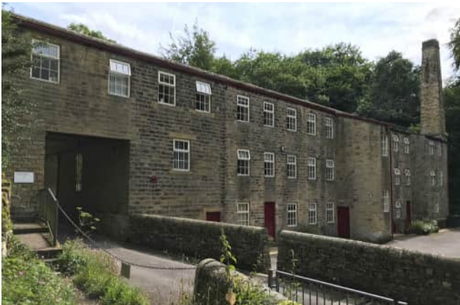
Grade II Listed Bents Mill, Hallas Bridge
