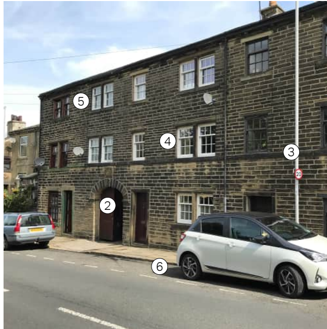
Photograph 5: Grade II listed former weavers' cottages, Main St
