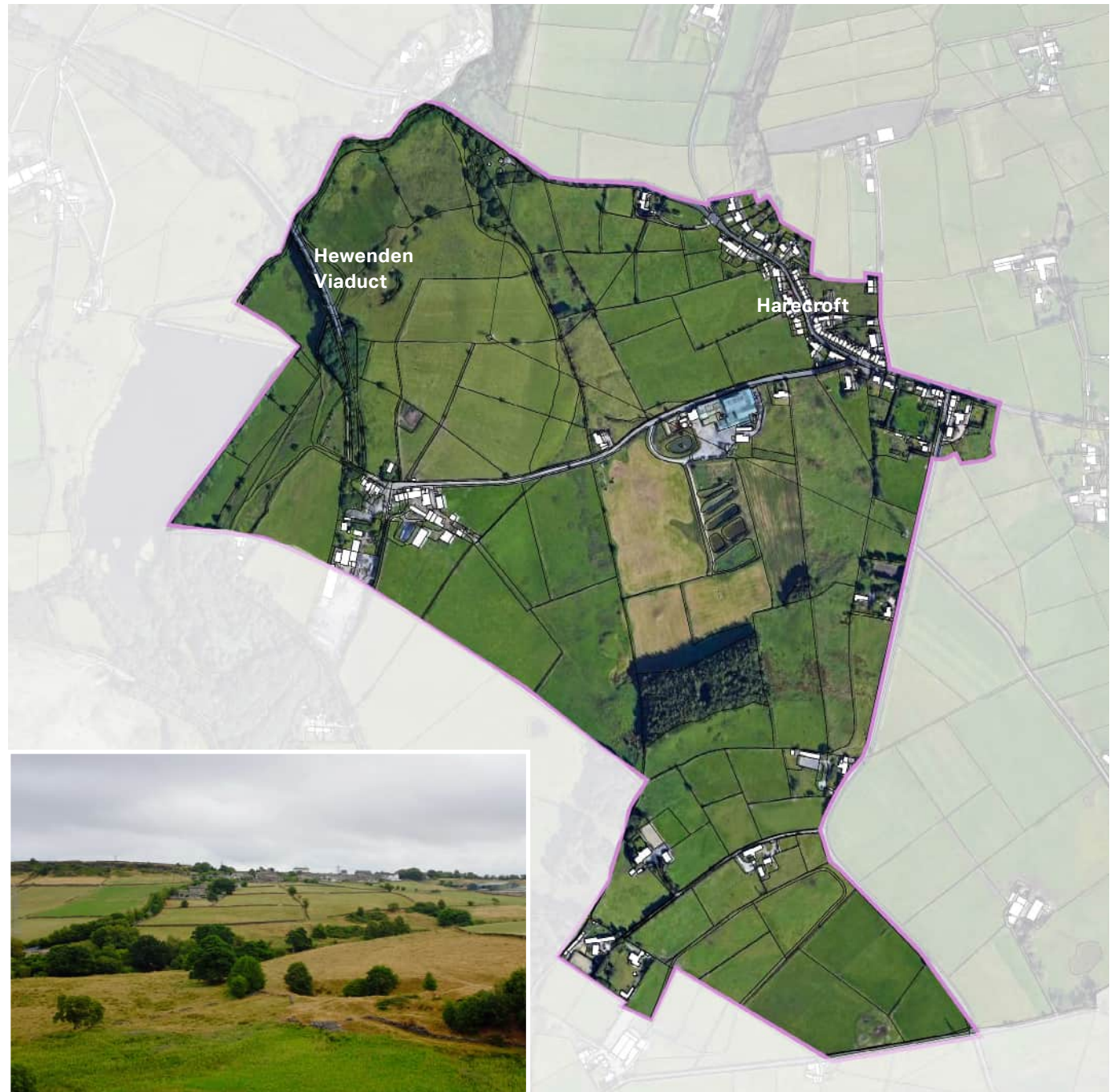
View from Hewenden Viaduct to Harecroft
