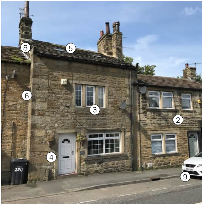
Photograph 1: Main St at Lingbob
