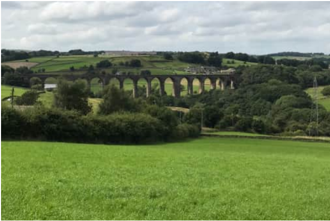
Grade II Listed Hewenden Viaduct
