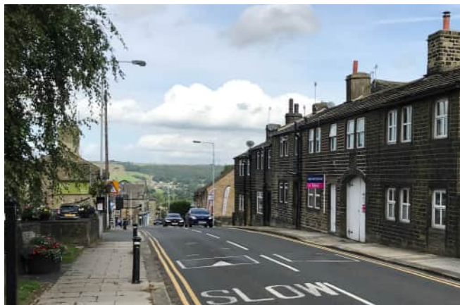
View 1 Looking north from Main Street
