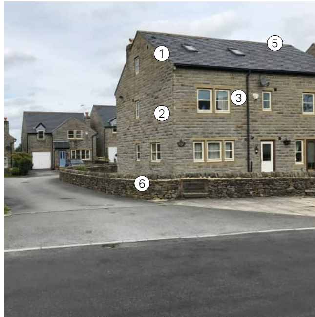
Photograph 20: Broomfield, Crack Lane
